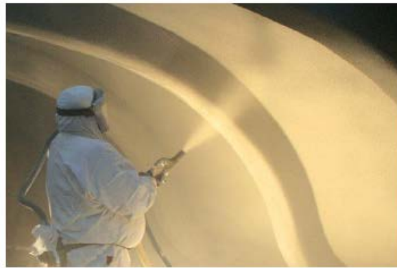
b) Spraying a fine grained concrete layer [20]
