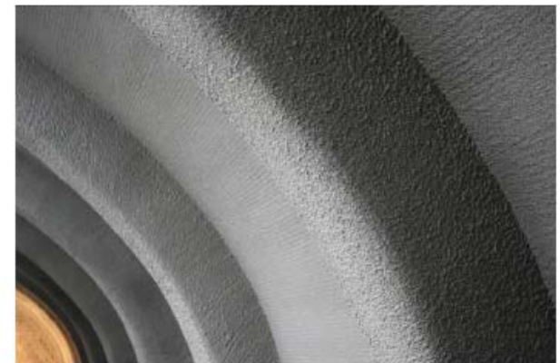
d) Ready TRC surface
