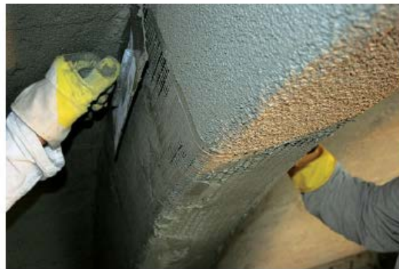
c) Application of carbon fabric into the fine concrete (right photo: [20])
