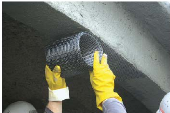
c) Application of carbon fabric into the fine concrete (right photo: [20])
