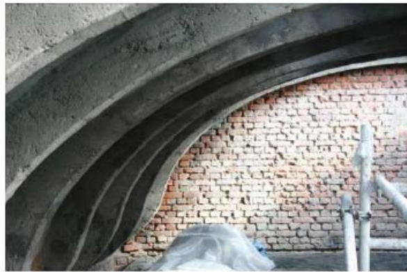
a) Prepared reinforced concrete structure
